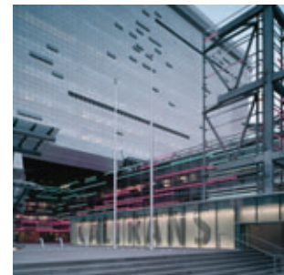
The Eli and Edythe Broad Plaza at Caltrans District 7 Headquarters in downtown Los Angeles
