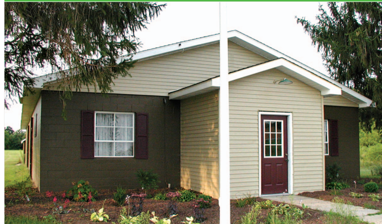
The San Pierre Lions Club received funding for new ceiling tiles for the Community Education Center.
